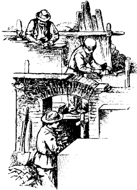
FIGURE 1.6 The foundation stone of your dissertation
